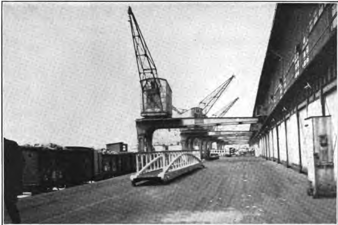
Dock at Hamburg (Use of Movable Cranes)
